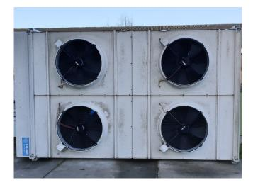
exchanges LU-VE S.p.A. Via Caduti della Liberazione 53 21040 Uboldo (VA) Italy Fully Electronically Tested HEAT EXCHANGER Code 30159977 XAV9X 8922 V/H EC 400 + IS CODE: 10127490 S/N: 412910/2013 PED CAT I Fluid: R22-R134A R407C-R404A-R507 Volume 87.00dm<sup>3</sup> Ts: -10°C +55°C Max Pres 3MPa VENTILATION Nr. Motors 4 Tens. 400V 50/60Hz  $\triangle$ 625W 1,1A X DEFROSTING -11-N° N°
